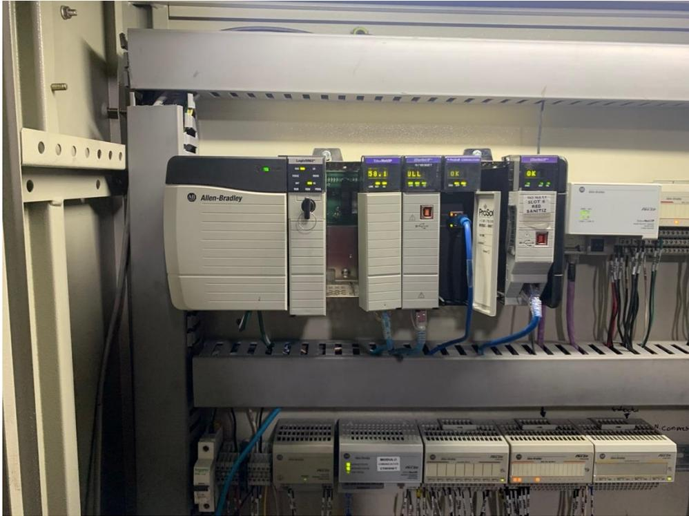
Figura 13. ControlLogix Allen Bradley.
